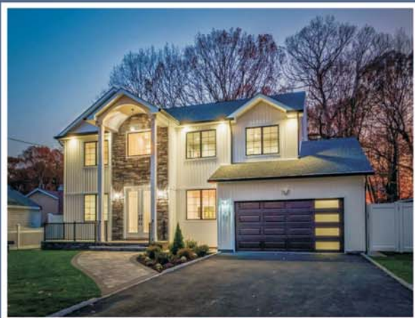
West Hempstead New Construction
